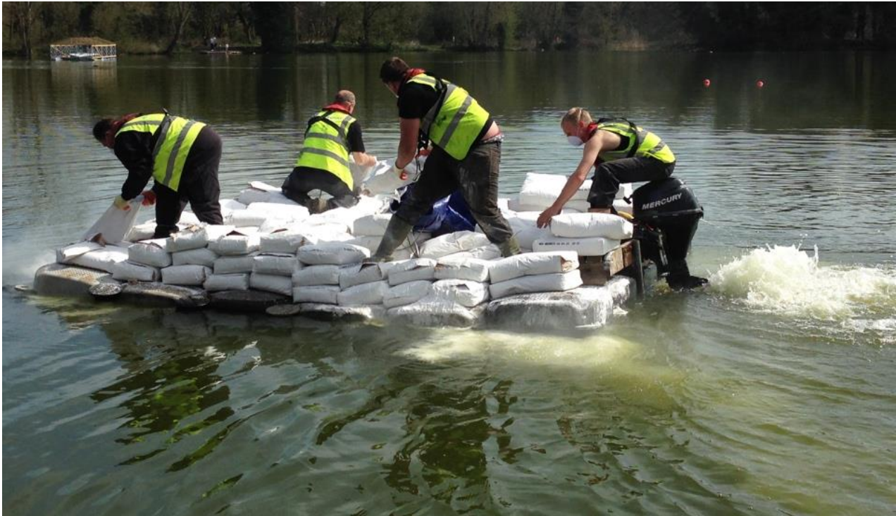
Plate 2. Installation of AquaBio.
